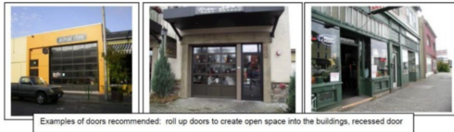
Figure 14.158-11: Recessed Doors, Contemporary Door Hardware, Single/Double Doors, Side Lites, and Transom Windows
