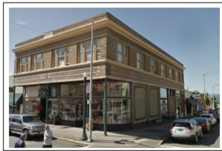
Figure 14.158-4: Base, Middle & Top of Building
