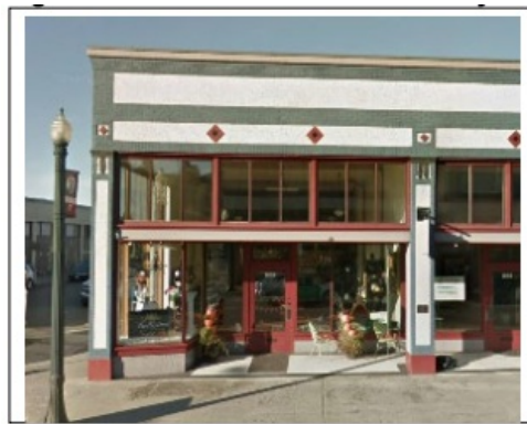
Figure 14.195-4: Prominent Main Entry
