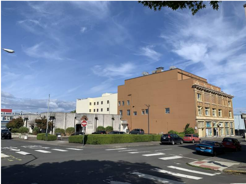
View looking northeast showing parking lot and adjacent buildings.
