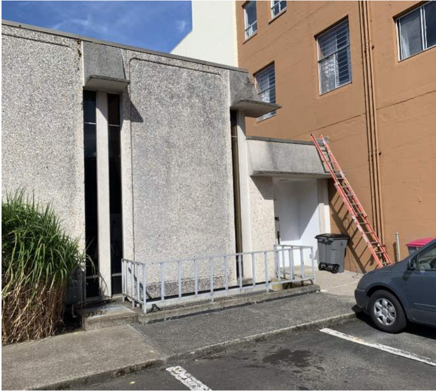
Secondary south staff entrance.
