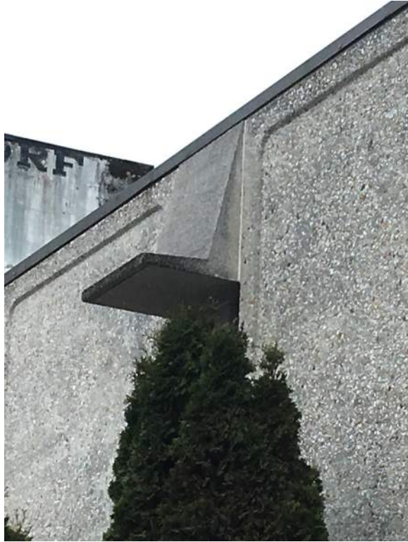
Typical cast stone eyebrow hood.
