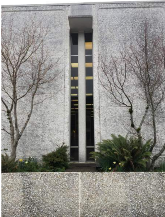
Typical paired gun-slit windows with cast stone column cover and eyebrow hood.
