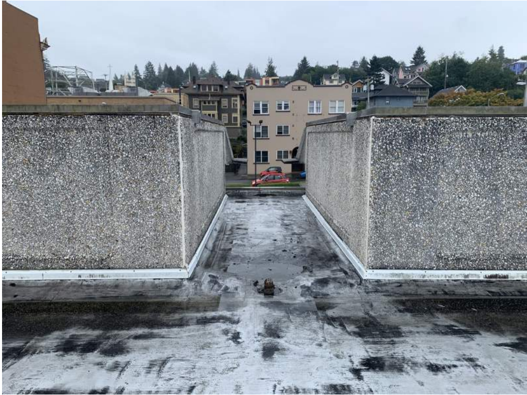
Typical roof conditions, view looking south.
