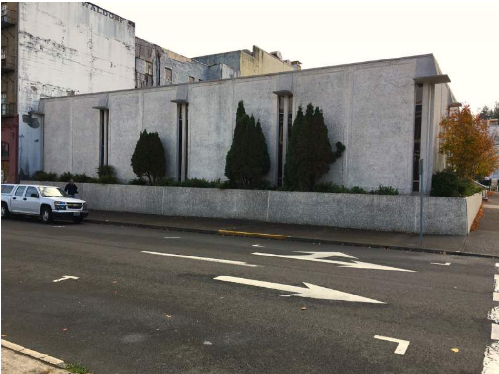
North elevation, planter, and sidewalk.
