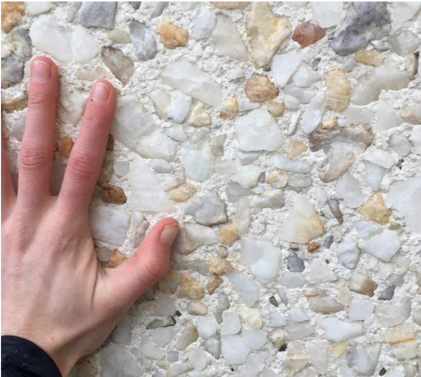
Close up of pre-cast concrete aggregate at clean area.
