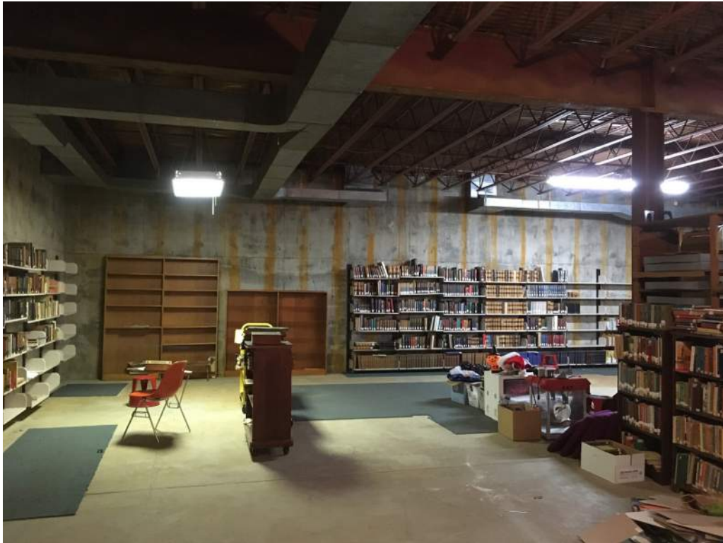
Unfinished, open basement space.
