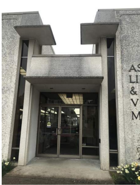
South public entrance.
