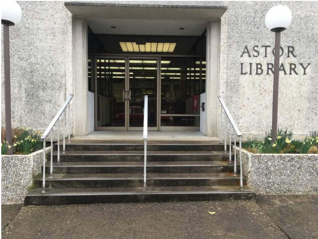
Primary/west entrance, stair, railings, and site lighting.
