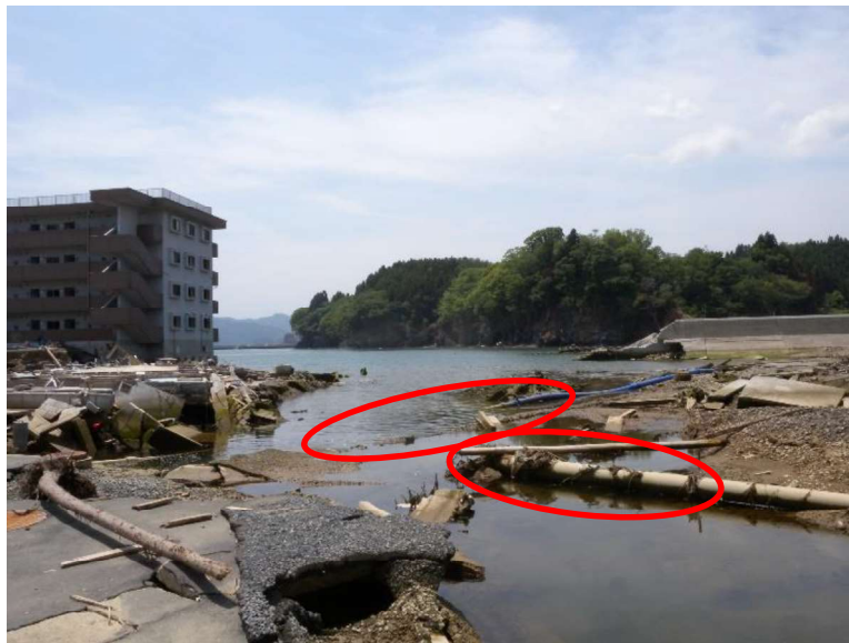
(b) Pipelines Exposed Adjacent to Road
