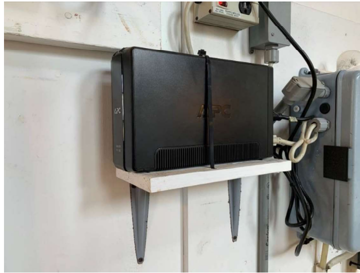
Figure 3.17 – Chlorination System Backup Battery not Adequately Restrained
