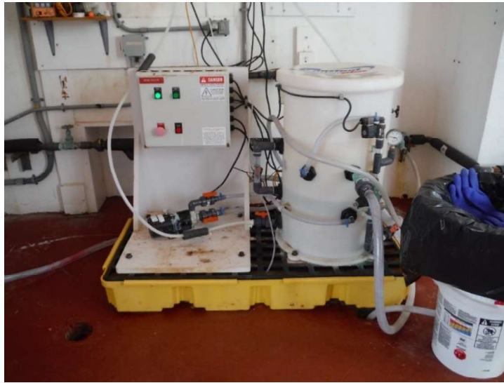
Figure 3.31 – Chlorination System and Spill Containment Skid not Adequately Restrained
