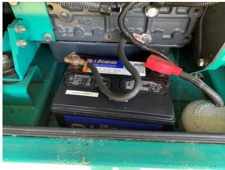
Figure 3.40 – Emergency Generator Starter Battery not Adequately Restrained
