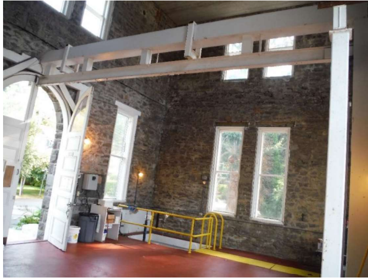
Figure 3.19 – Crane Rail System (no longer in use)
