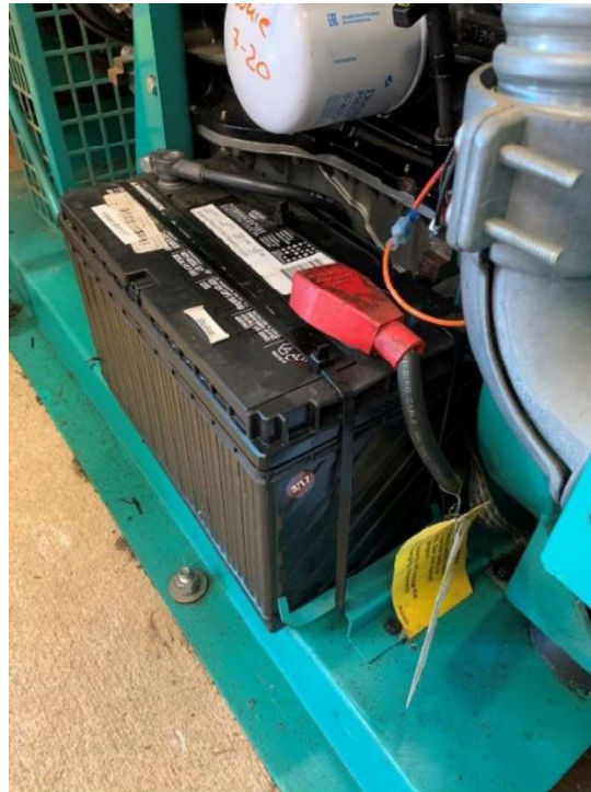
Figure 3.48 – Emergency Generator Starter Battery not Adequately Restrained
