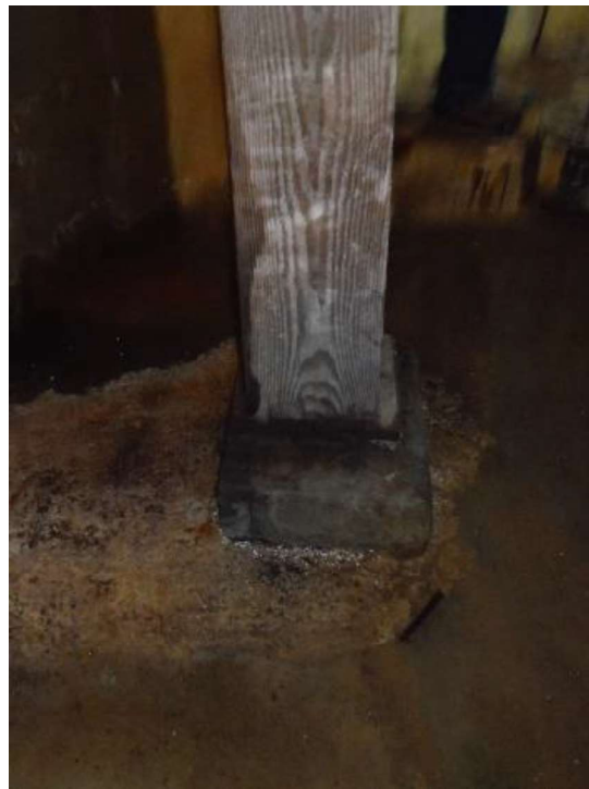
(b) Post to Slab-on-Grade
