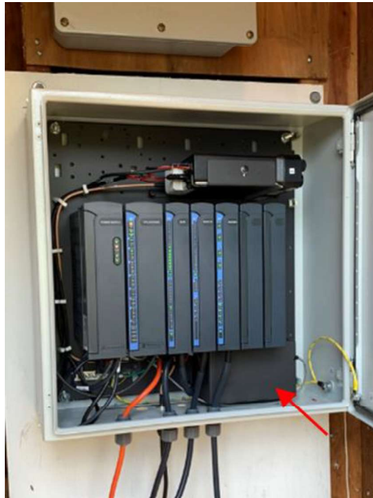
Figure 3.38 – SCADA Backup Battery not Adequately Restrained
