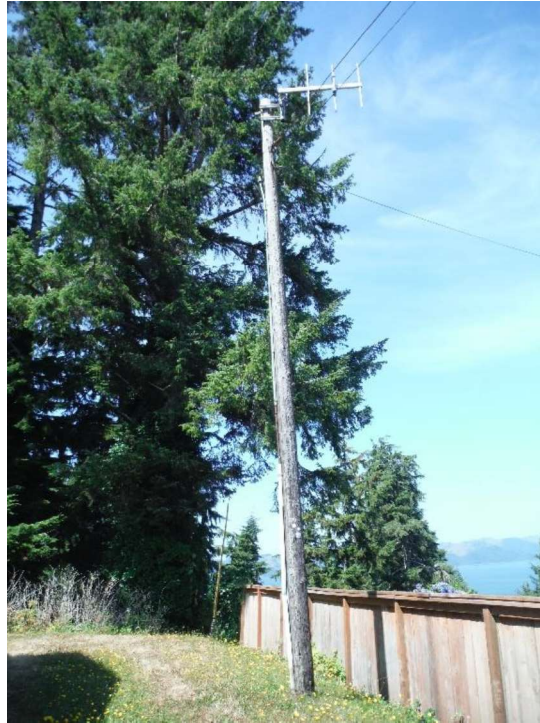
Figure 3.47 – SCADA Antenna Attached to Wood Pole
