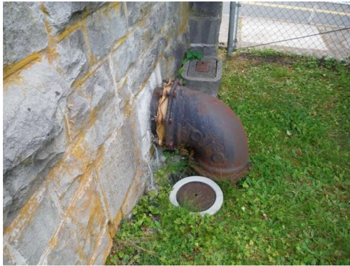
Figure 3.11 – Reservoir Inlet Pipe Penetrating Gate House Stone Masonry Wall without Adequate Flexibility
