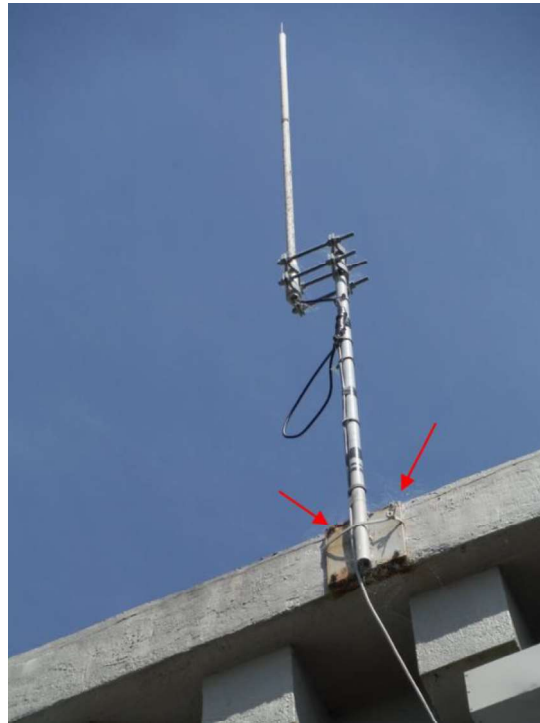
Figure 3.39 –SCADA Antenna to Roof Slab Connection with Potentially Inadequate Edge Distance for Concrete Anchors
