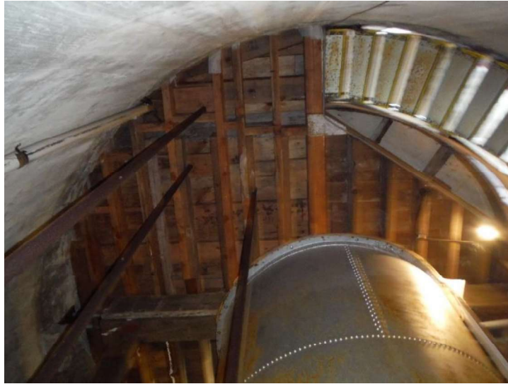
Figure 3.8 – Straight-Sheathed Wood Diaphragm
