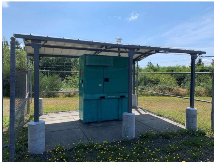
Figure 3.27 – Reservoir 3 Gate House Emergency Generator
