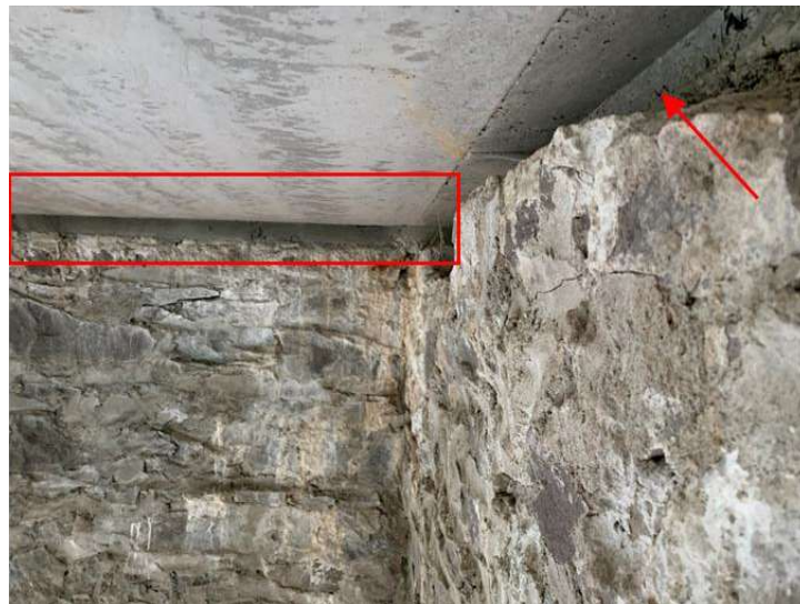
Figure 3.7 – No Evidence of Positive Connection Between Concrete Roof Diaphragm and Stone Masonry Walls
