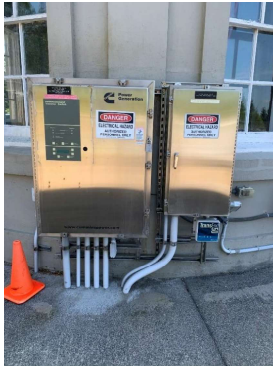
Figure 3.36 –Conduits from Below Grade Connecting to Electrical Cabinets without Flexibility
