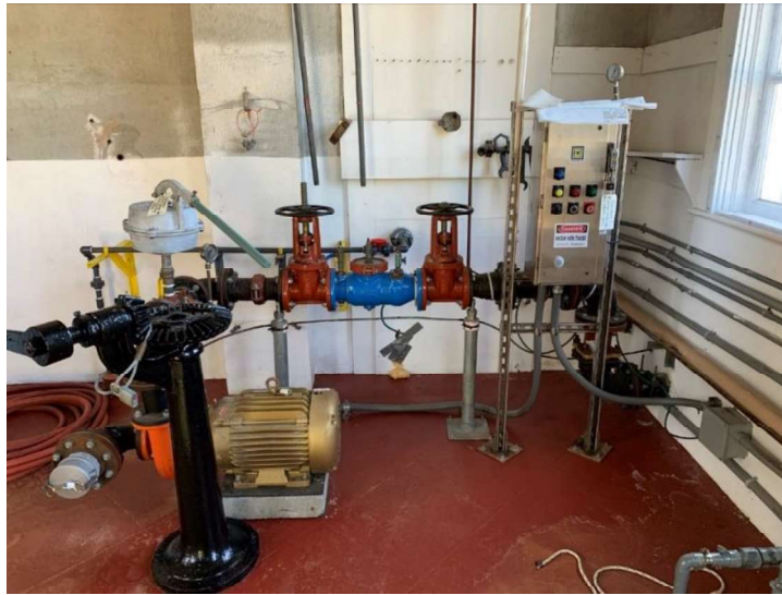
Figure 3.35 – Pumping System Used to Clean Reservoir Cover not Adequately Braced
